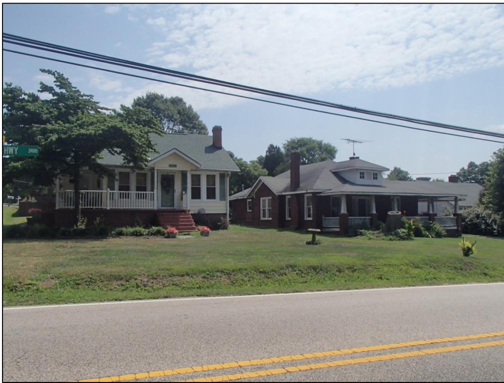
Figure 25: Bungalows on Kannapolis Highway
