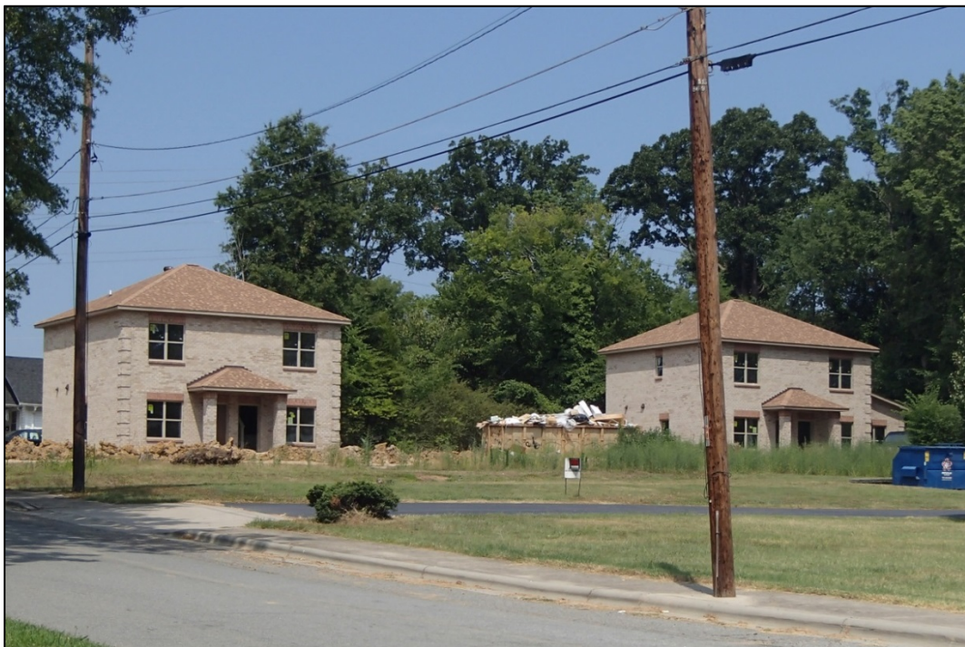
Figure 29: Townhouses under construction on Mills Avenue
