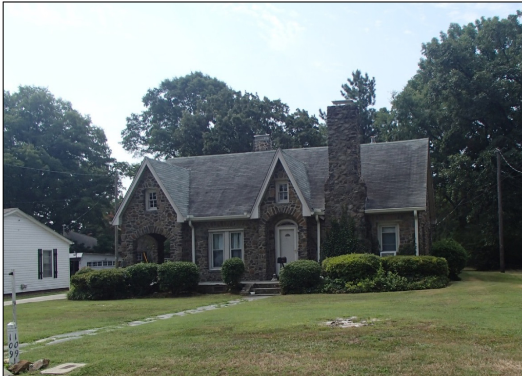
Figure 7: English cottage at 109 Maple Avenue
