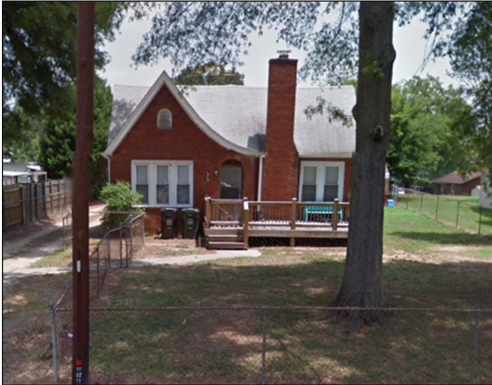
Figure 8: English Cottage at 1215 Central Drive
