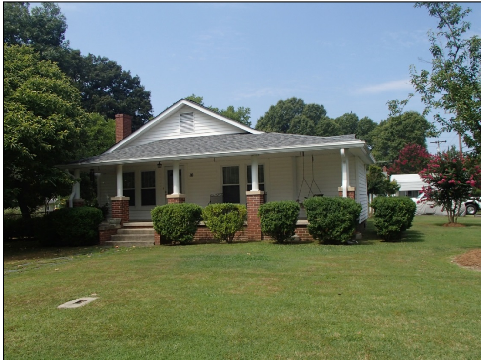
Figure 13: Bungalow on Willowbrook Drive
