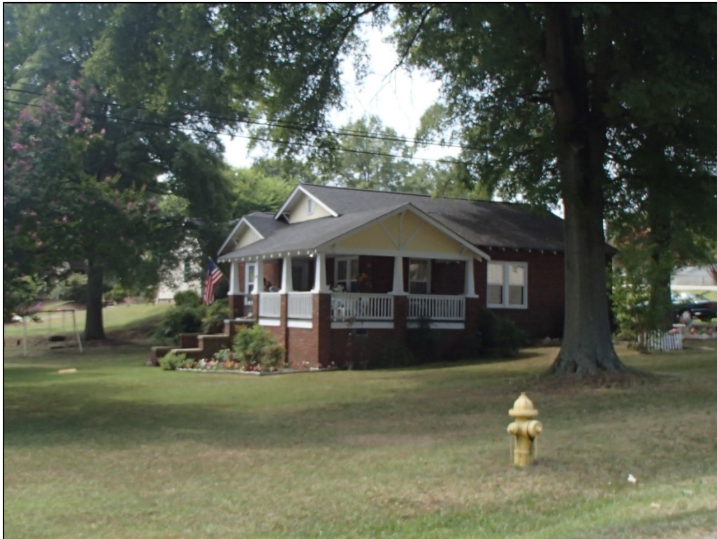
Figure 5: Bungalow at 2402 Kannapolis Highway at the corner with Willowbrook Drive
